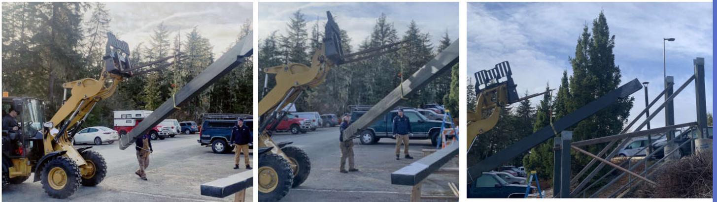
These pics above are from the construction of the covered stairs at Student Housing. Donny Sims, (mechanic) is operating the forklift and Dusty Rautiainen (carpenter), is directing the placement of the beams while Dana Wade (plumber), is handling the tag line.
